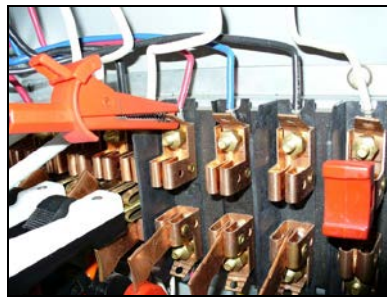
Open potentials (if driving voltage). Move alligator clips to top
